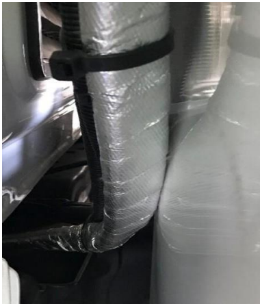
Figure 1.20: Hose Rub (NOT ACCEPTABLE)
