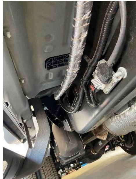
Figure 1.7: Hoses Routed Under Vehicle
